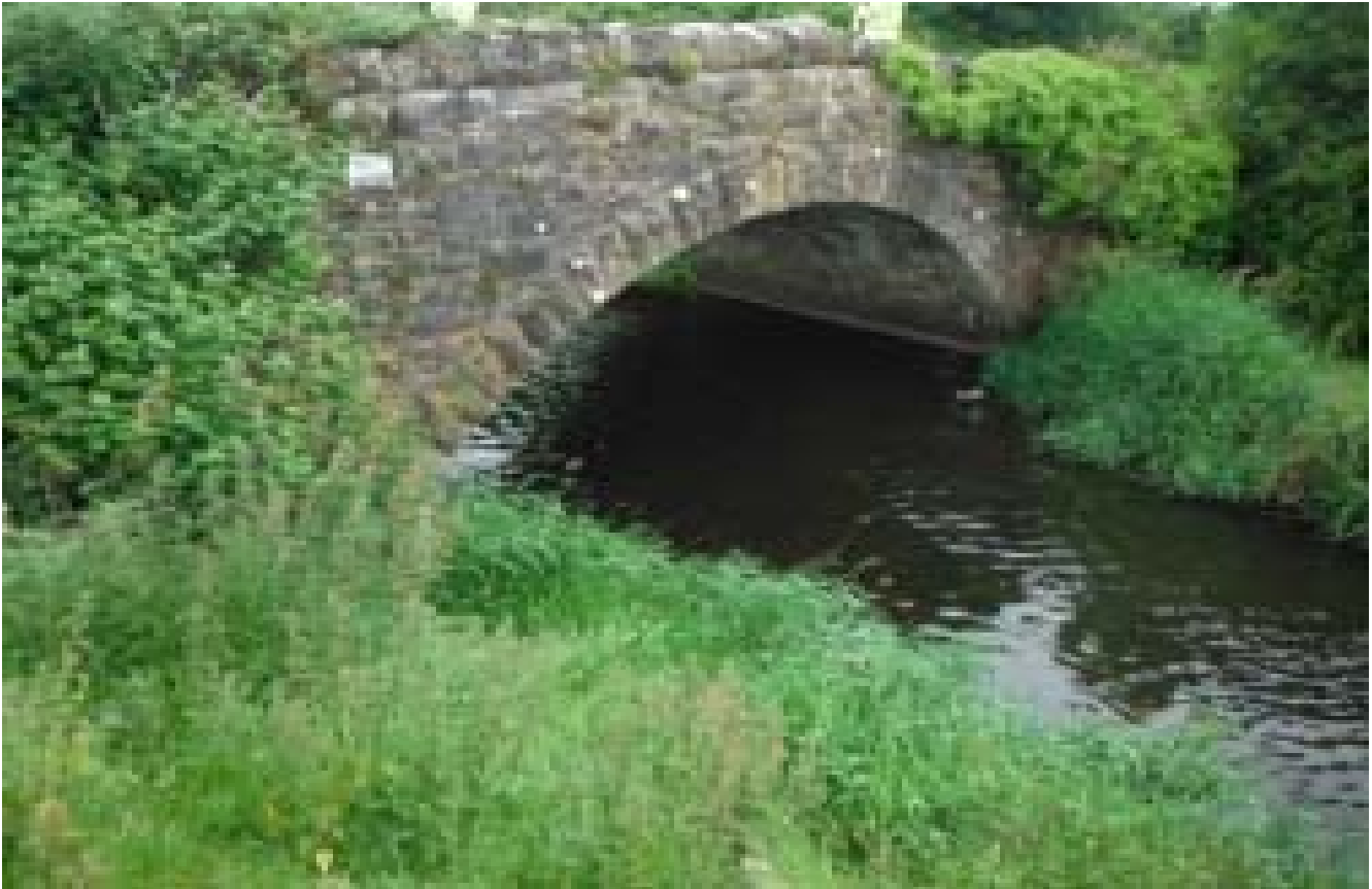
Figure 9.6: Slate River crossing at Agar Bridge
